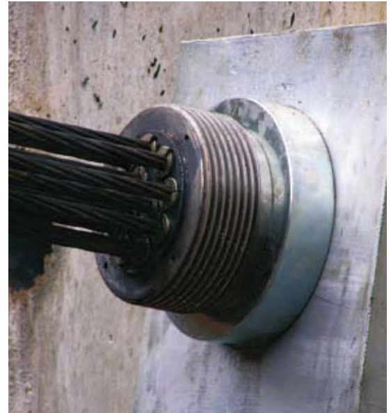
Anchor Head Detail
