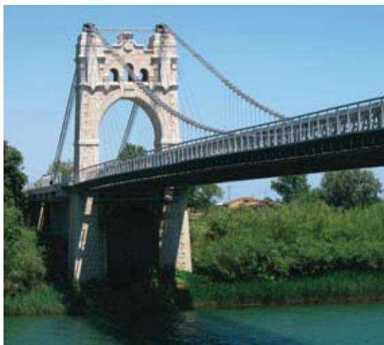
^ Amposta Bridge (Spain)
