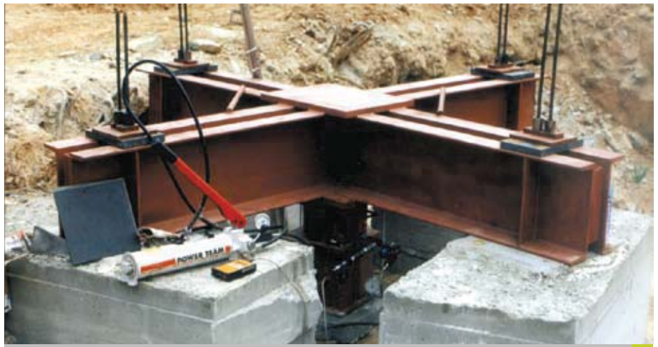
Test Load on a High Speed Railway Viaduct (Spain)
