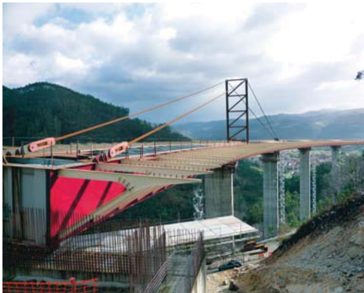
^ Regueiron Bridge (Spain)
