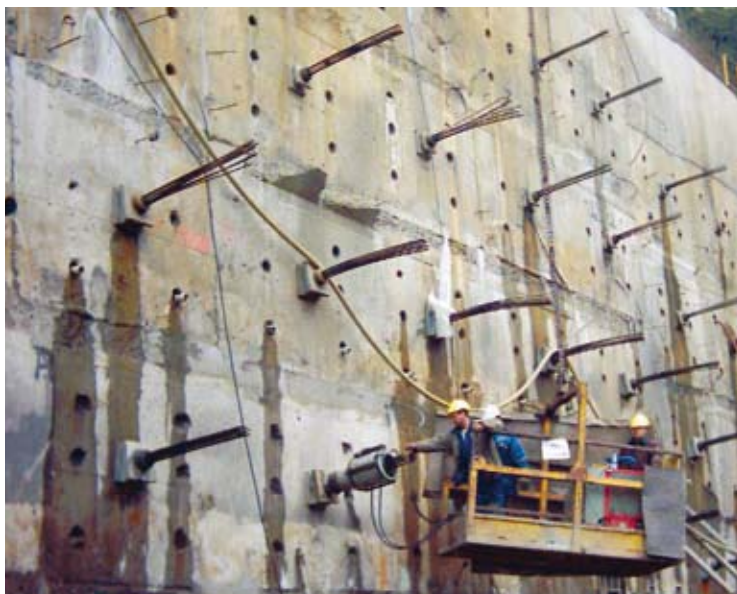
Ground Anchor Installation
