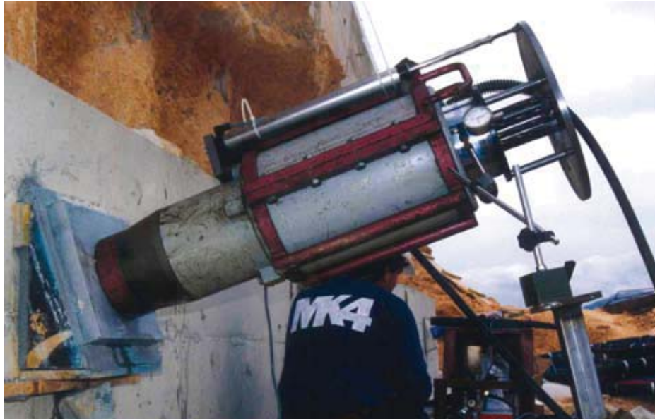
Ground Anchor Stressing
