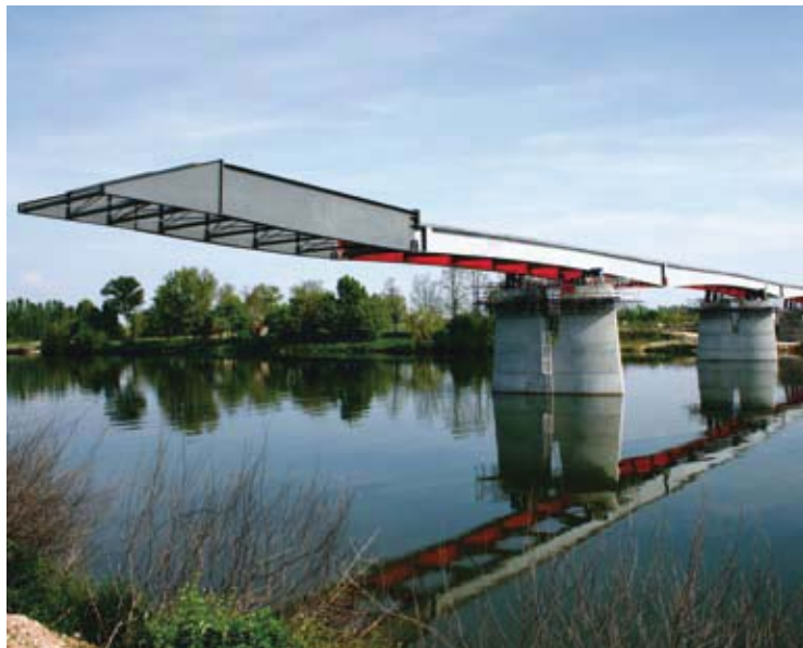
Tarn Viaduct - Moissac (France) ^
