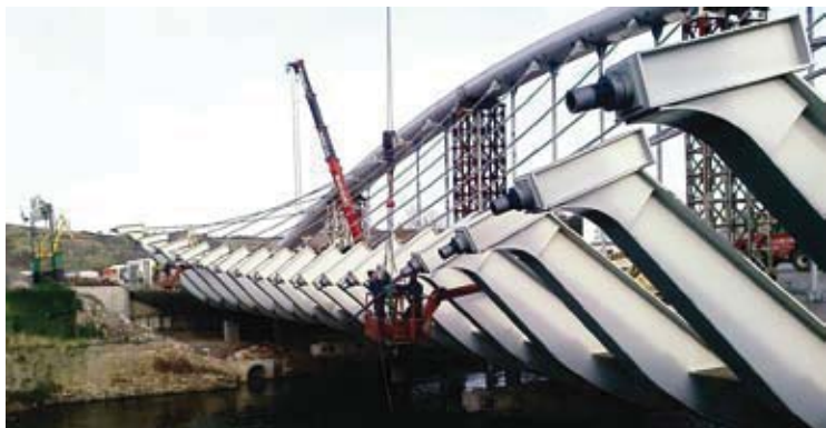
^ Galindo Bridge - Vizcaya (Spain)
