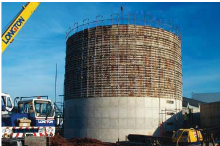
^ Market Dyrton Water Tanks (UK)
