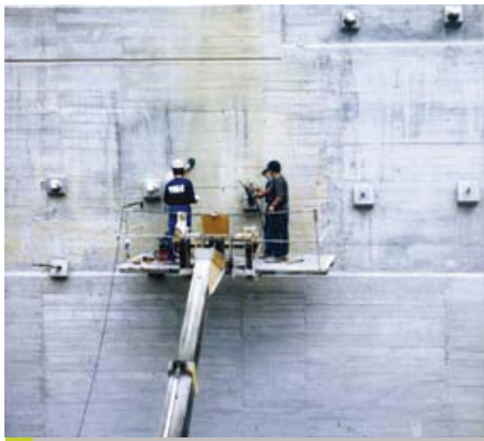
Ground Anchor Replacement
