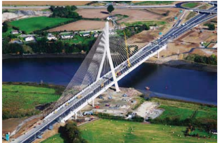
Waterford Bridge (Ireland) ^
