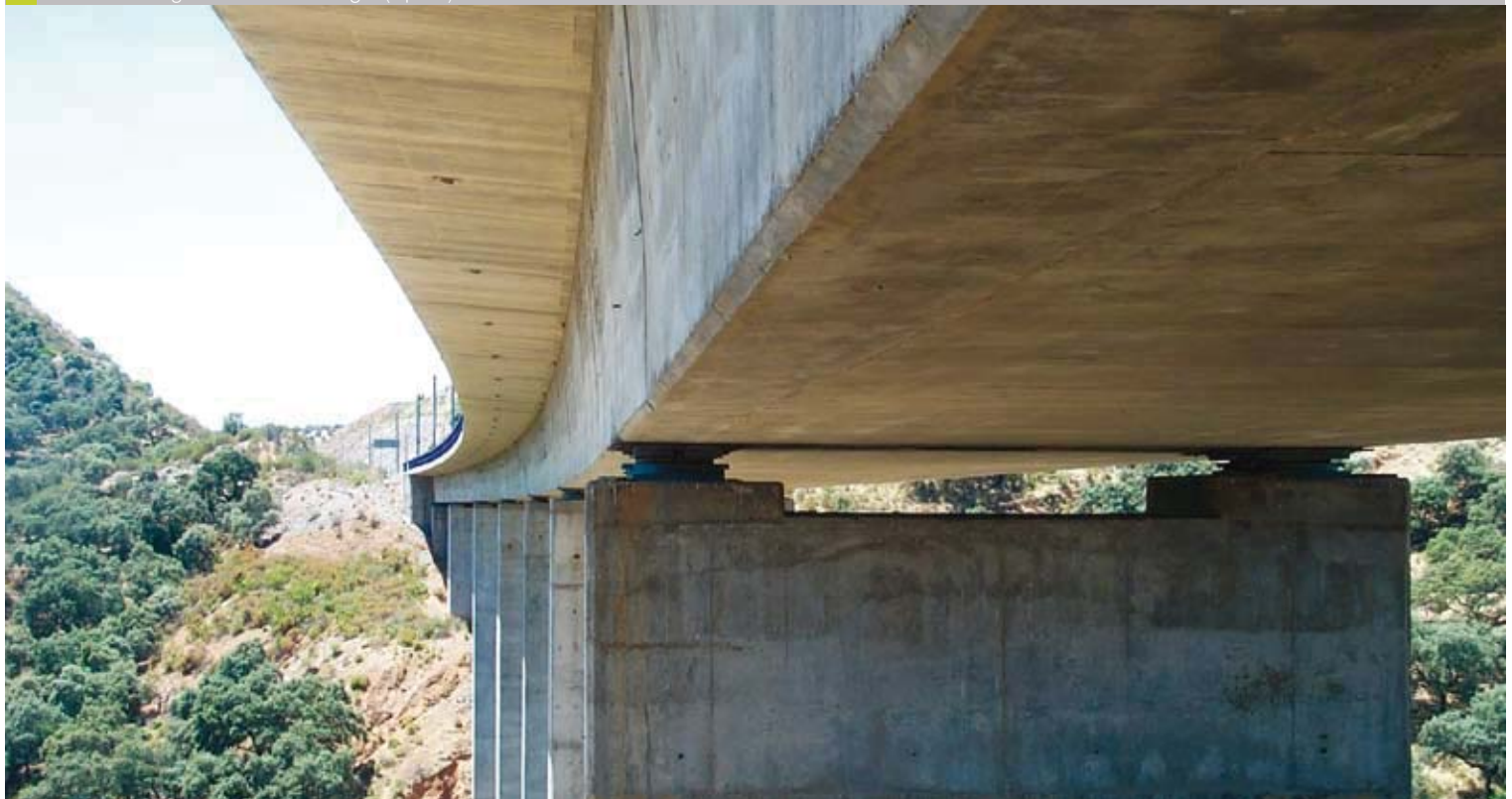
^ POT Bearings on a TGV Bridge (Spain)
